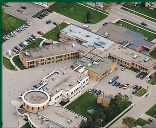
Aerial view of Hospital and Wellness Centre: Maurice Oliver photograph
